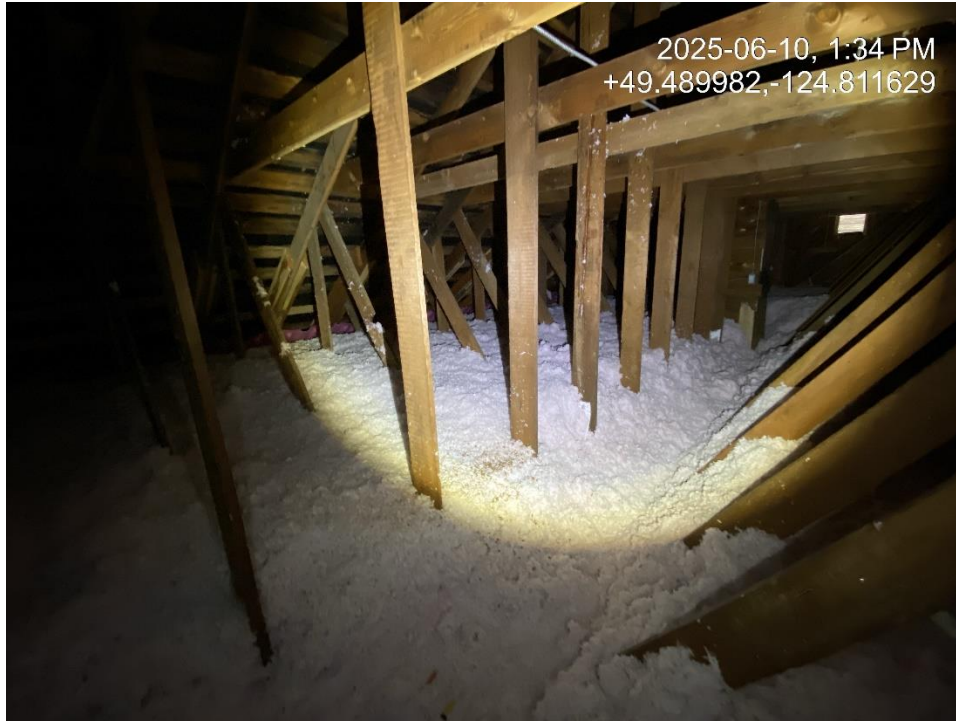
Figure 6 Roof framing over the main hall
