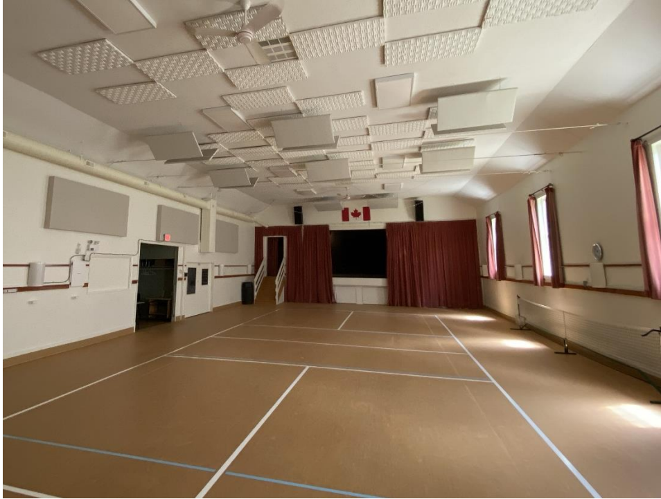
Figure 10 Main hall with steel cable tension ties
