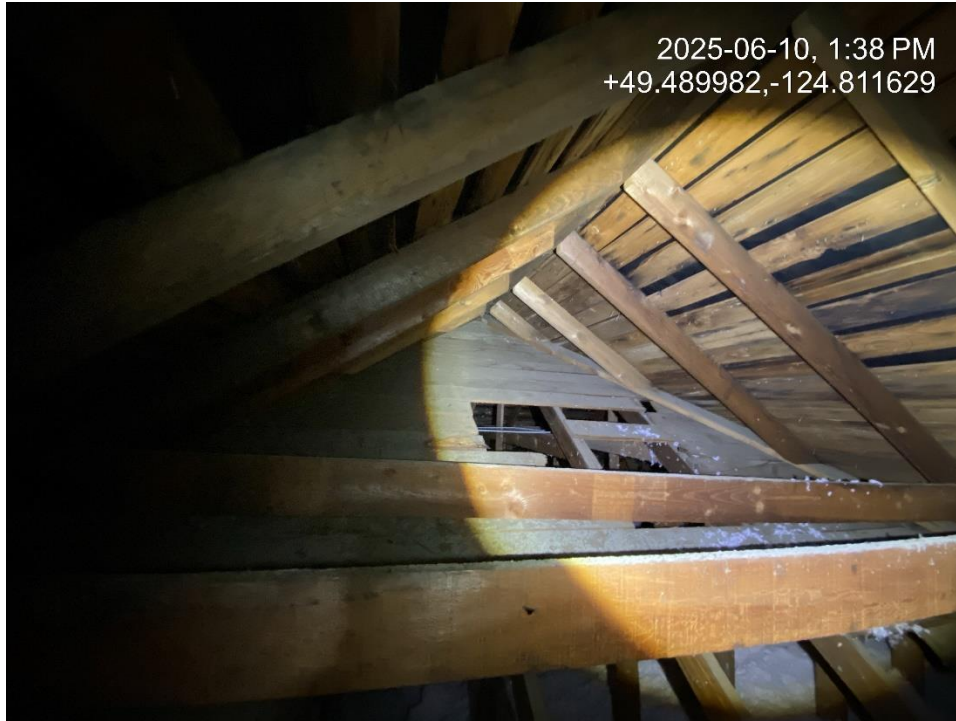
Figure 8 Intersecting roof framed on top of main hall roof framing
