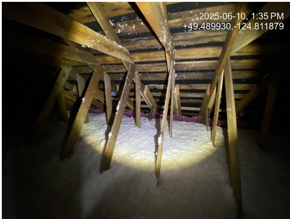
Figure 7 Roof framing over the main hall with sistered rafters along lower eaves
