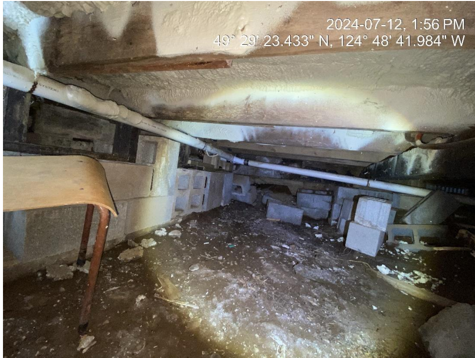
Figure 16 Masonry rubble wall below the kitchen
