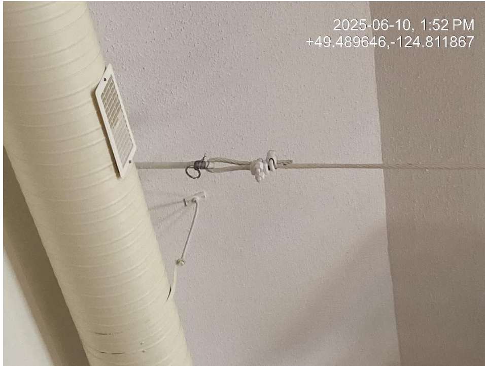
Figure 12 Tension tie to eye-bolt connection
