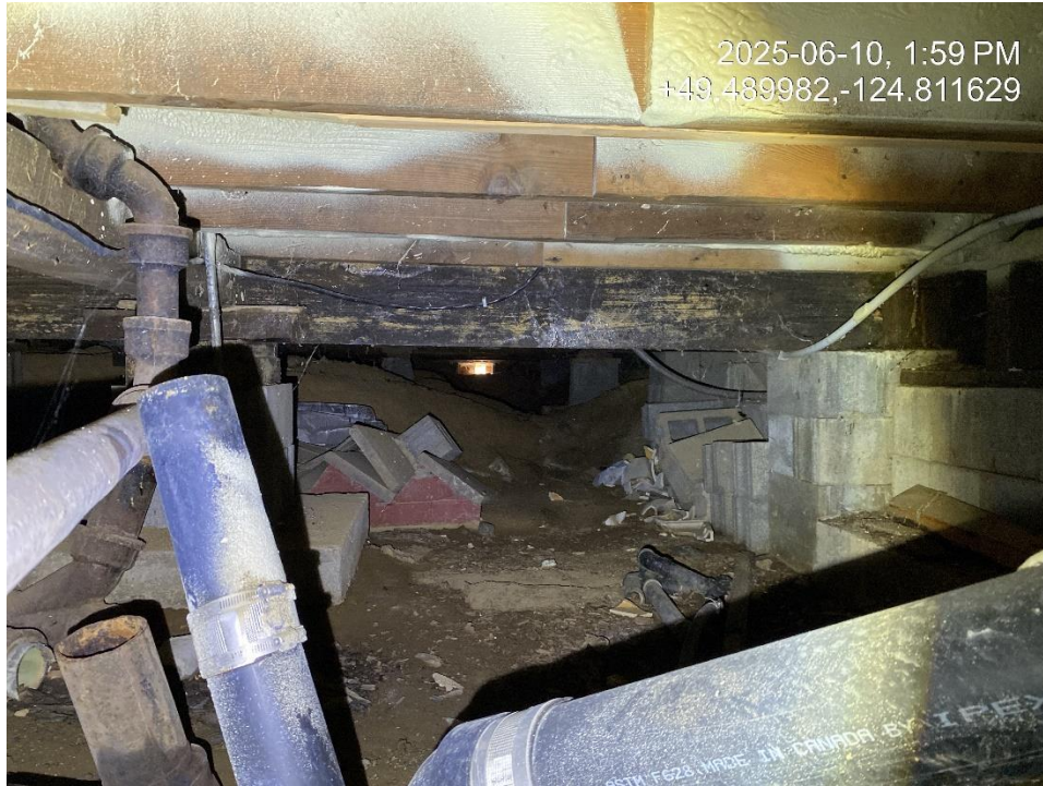
Figure 14 Floor beam and masonry supports
